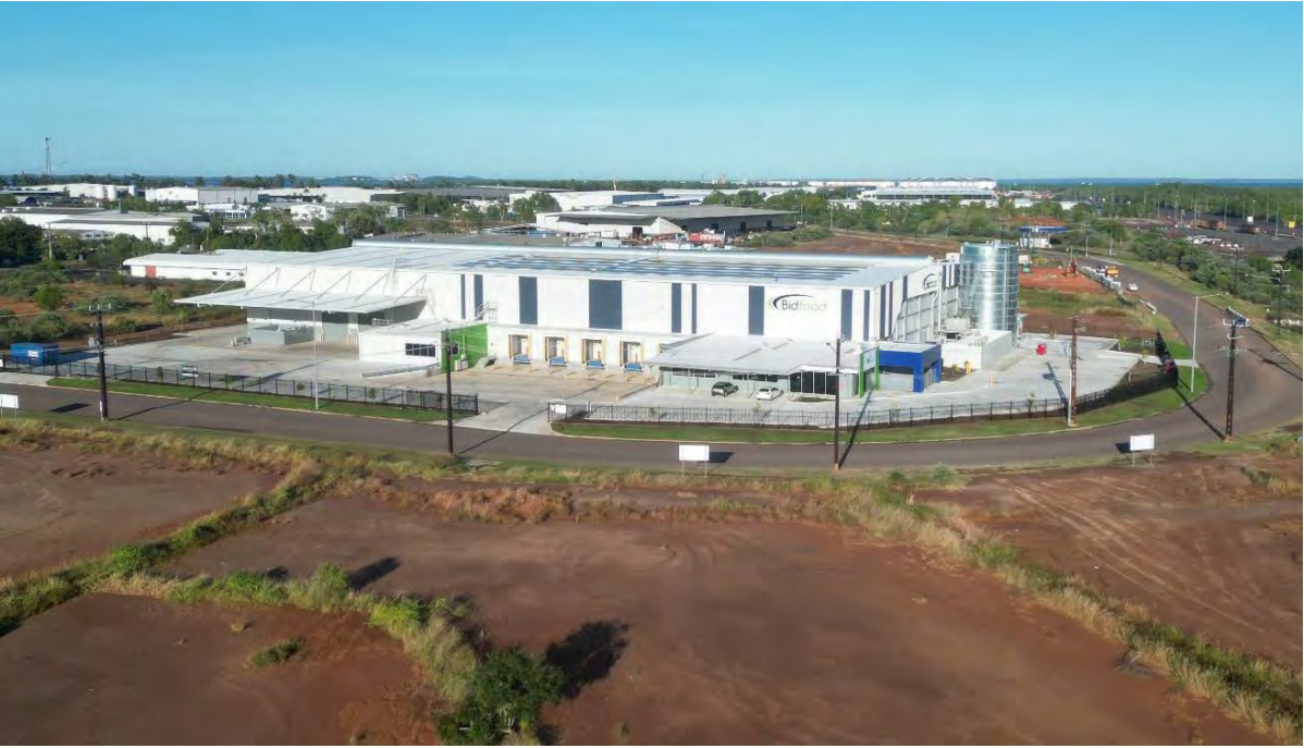
Bidfood's new facility, Darwin Business Park
