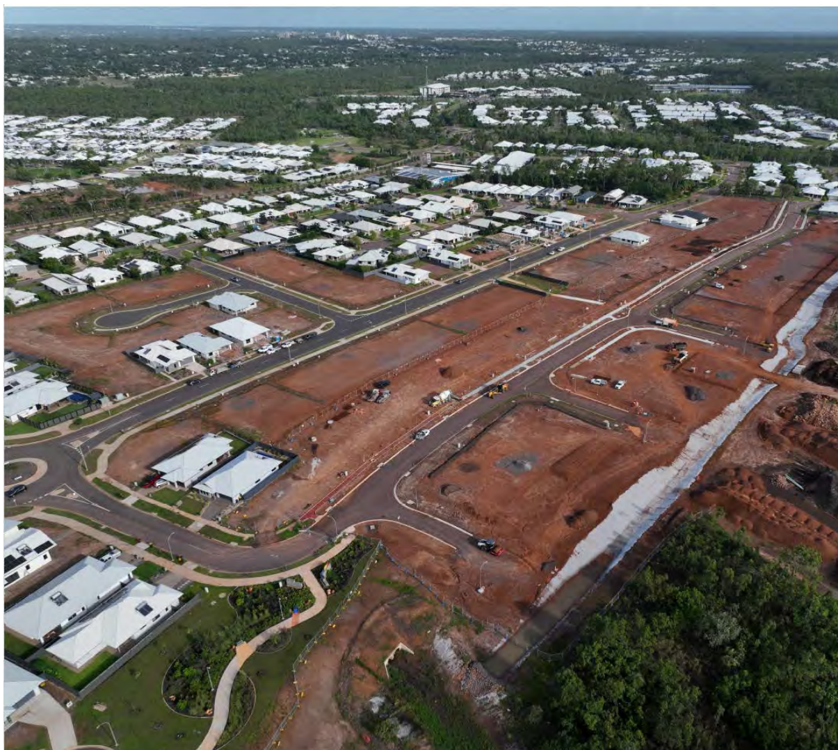
Phase 3.8 in final stage of construction – January 2024
